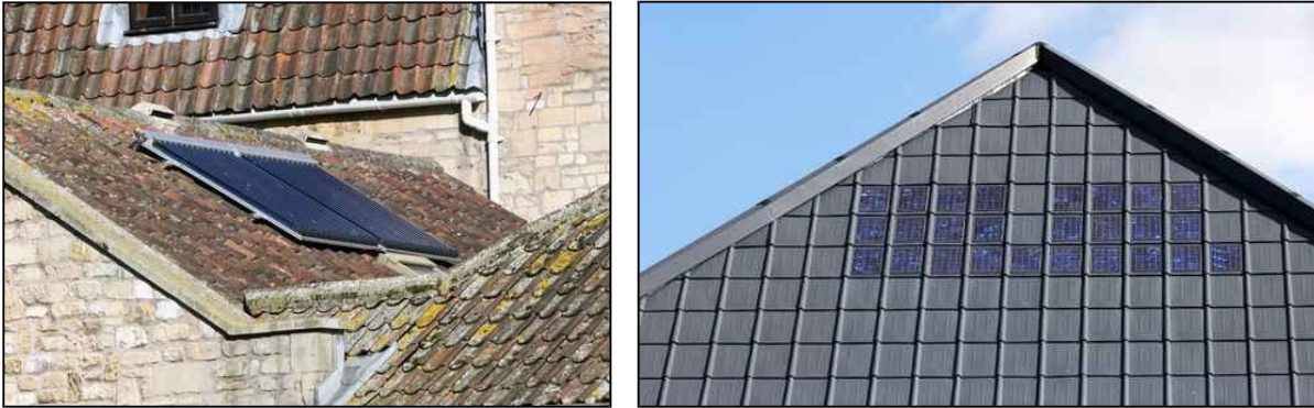
Figure 3: a) Discreetly located solar panels on historic buildings and b) solar roof tiles
