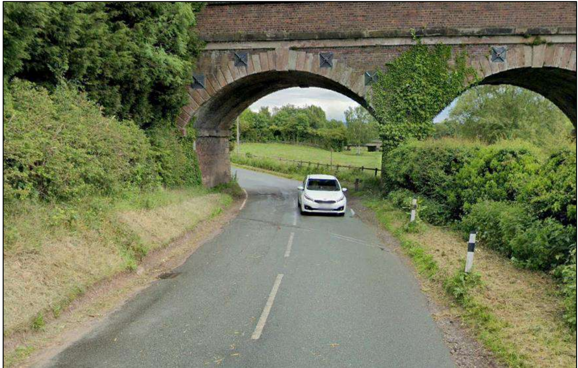
Figure 9. Penkridge Railway Viaduct
