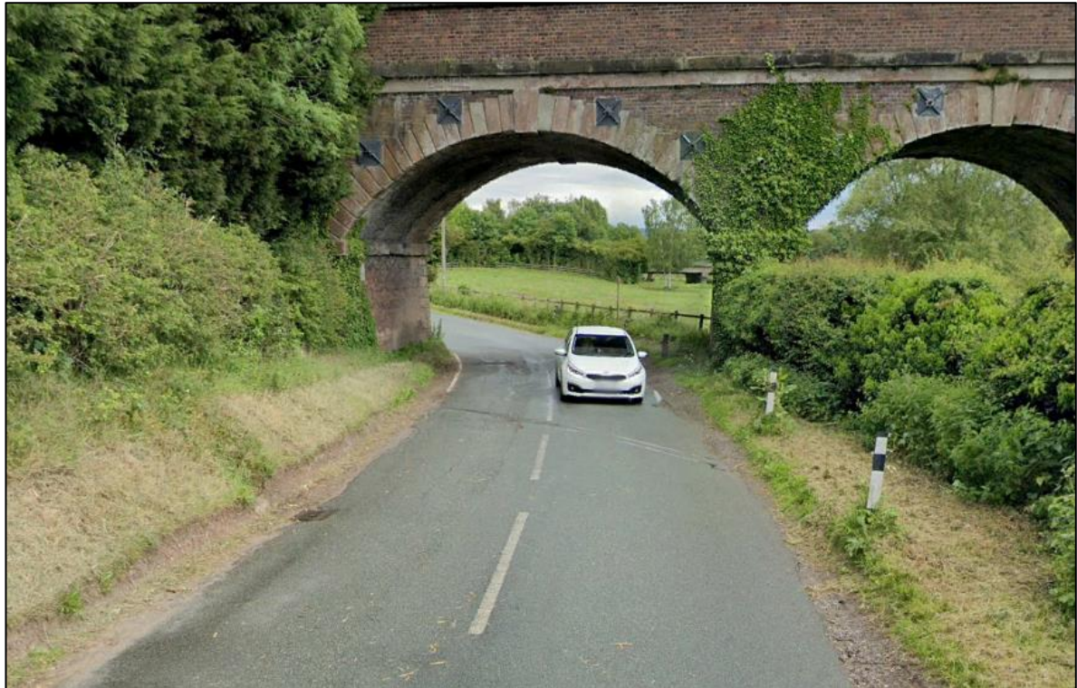
Figure 9. Penkridge Railway Viaduct
