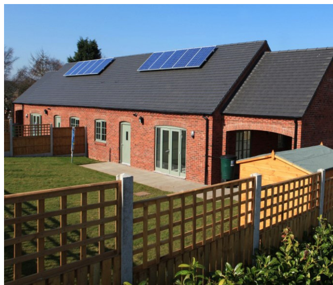
This development on Himley Lane, Swindon, uses the traditional farmstead layout - common in South Staffordshire - whilst creating contemporary homes with high energy performance and modern materials.
