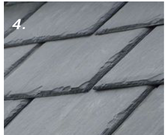
4. Blue-grey Welsh slate is also common across the district. Slate is lighter, more durable and weatherproof than clay. The colour can vary subtly from dark blue/grey to purple/grey.
