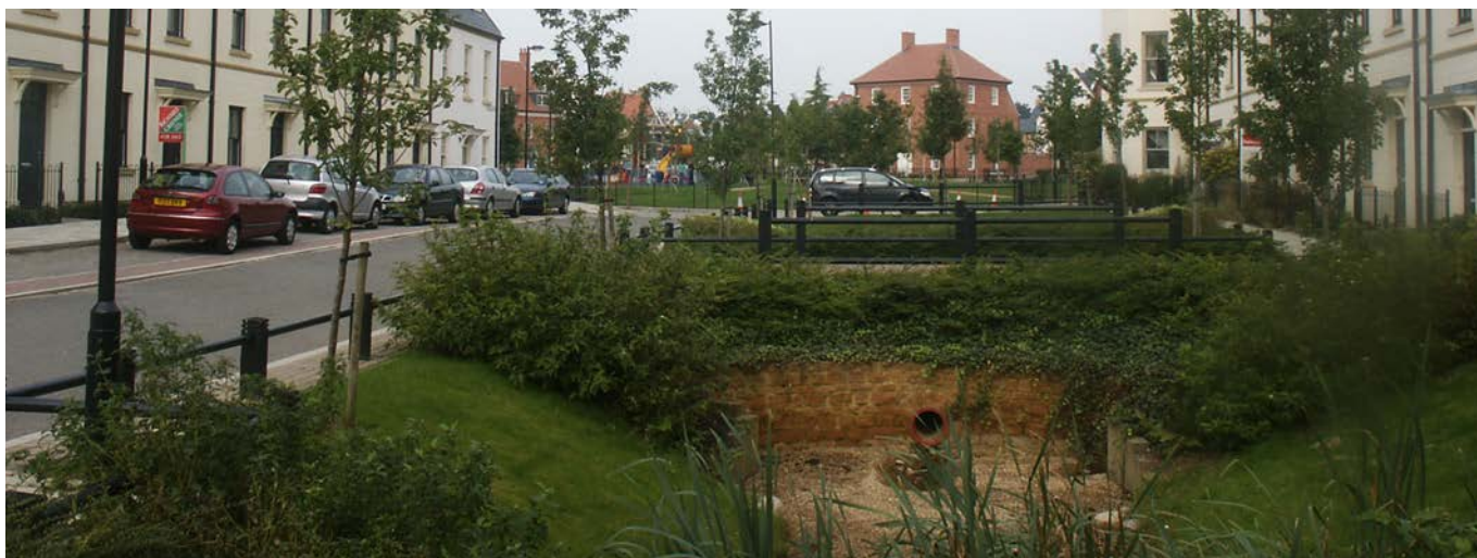
This artificial swale and channel has been designed to manage surface water run-off and provides an attractive and functional addition to the street.
