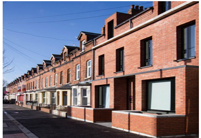
This modern infill development respects and continues the rhythm of the existing street.
