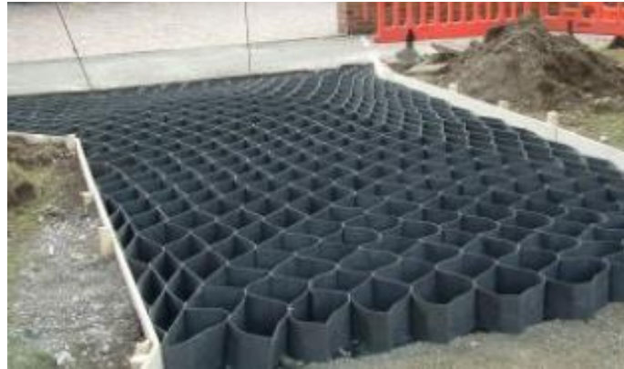
Figure 6: Cellular Confinement System Example
