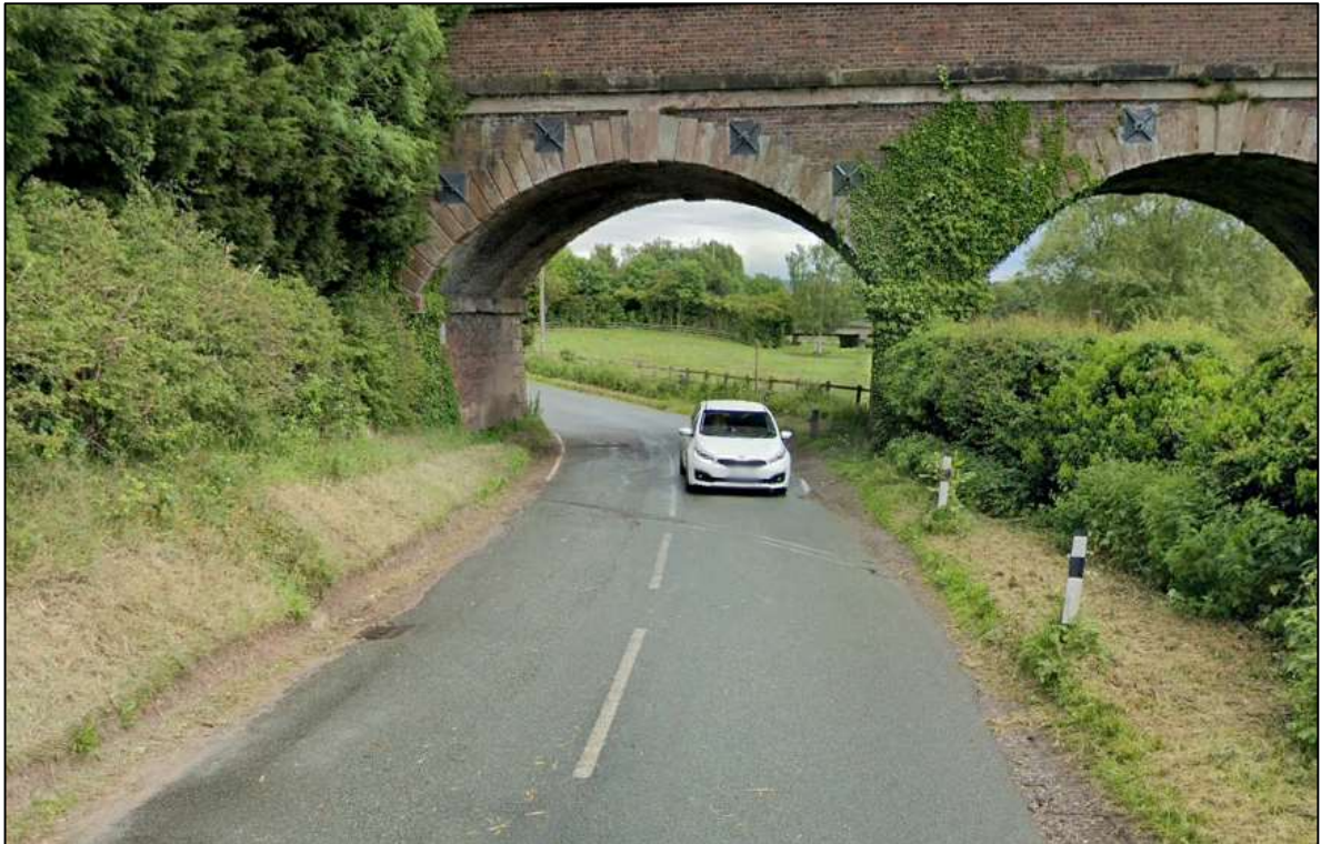
Figure 9. Penkrige Railway Viaduct
