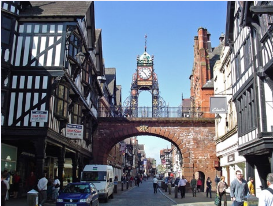
Eastgate Street, Chester. The original entrance to the Roman settlement and forms part of the city wall. The main part of the gateway is constructed from Triassic sandstone from the Helsby Sandstone Formation, which was also used to face the city wall.
